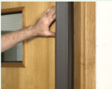
1 Secure the 'L' shaped end to door butting up to the back of the hinge.
